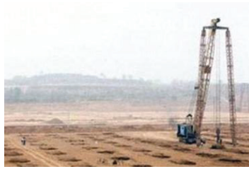
Fig. 5 (a): Construction example of dynamic compaction.
