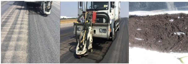
Fig. 1: Runway with deposited rubber and collecting sample using track jet.
