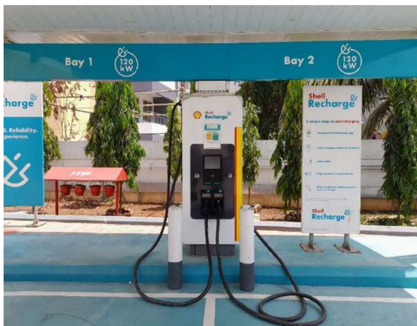
Fig. 3: 120 kW DCFC with 2 CCS 2 ports.
