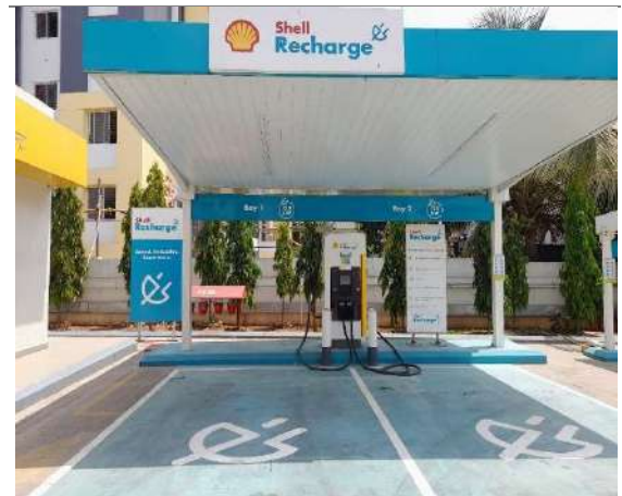
Fig. 2: 3.3 kW AC Chargers for 2-wheelers and 3-wheelers.
