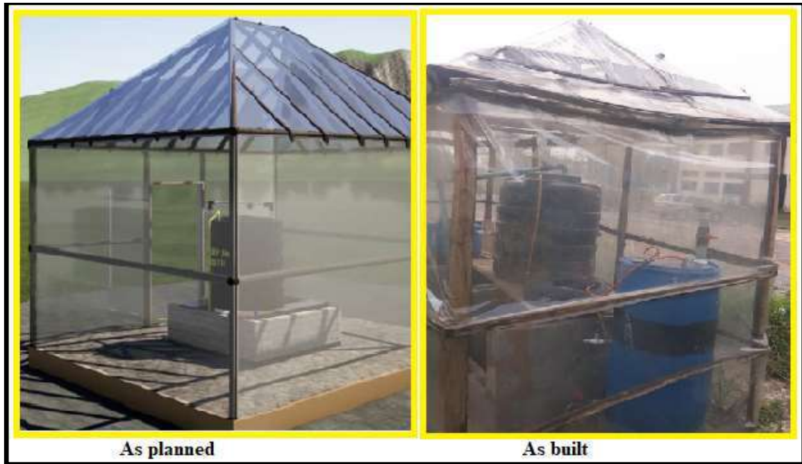
Fig. 2: Greenhouse for raising an anaerobic bio-digester.
