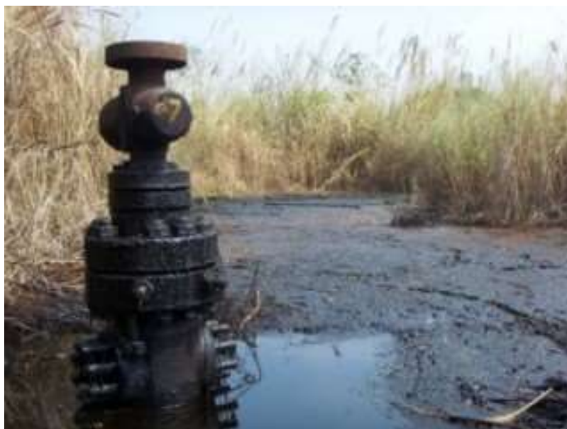
Fig. 1: Oil spillage in Nagaland.
