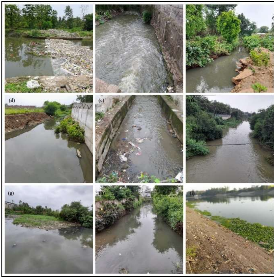
Fig. 4: Images of some informal urban drains sampled in the present study.
