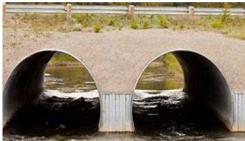
Fig. 7: Culvert under a roadway.
