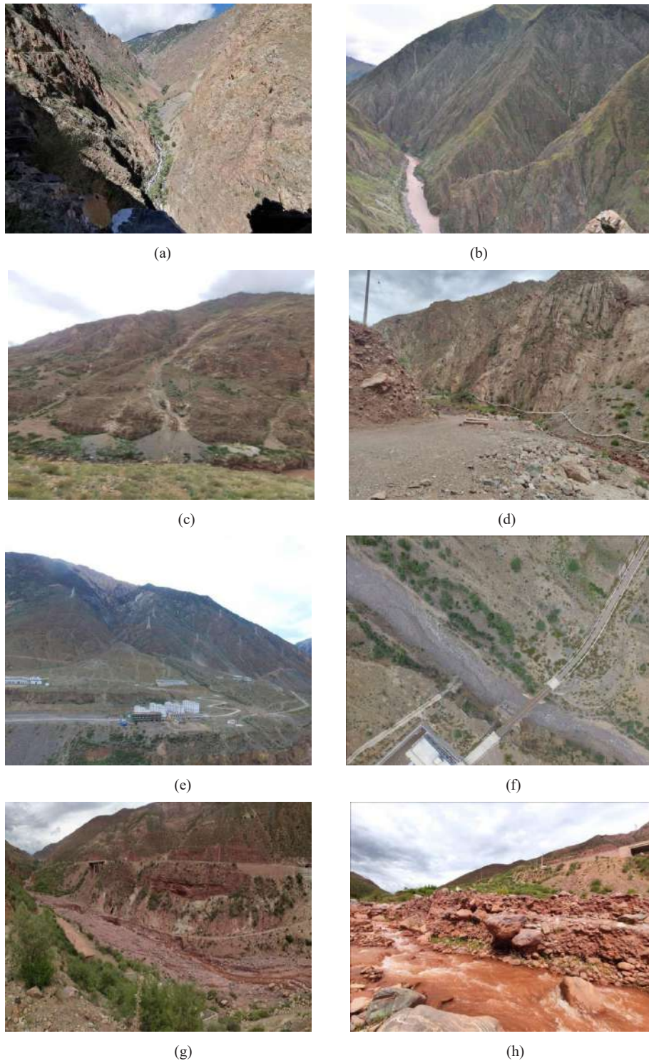
Fig. 2: (a) and (b) are the Rongsong debris flow gully channel form and Rongsong debris flow gully upstream left bank view, respectively. (c) shows the remote view of the left bank downstream of the No. 2 debris flow gully mouth at 400 m upstream of the dam site. (d) is the gully mouth of Duiba debris flow gully and the bedrock on both sides. (e) and (f) are the remote views of the old debris flow accumulation fan in Zhuka No. 1 gully and the natural 'drainage groove' on the old debris flow accumulation fan in Zhuka No. 1 gully, respectively. (g) and (h) are the panorama of the main channel of the Rongqu debris flow gully and the accumulation thickness of the main channel of the Rongqu debris flow gully, respectively.
