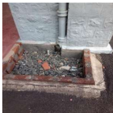
Fig. 3. Rainwater harvesting system
