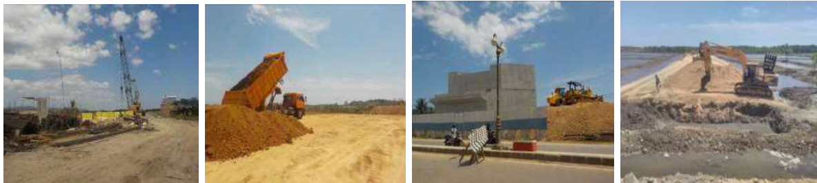
Fig. 2: Activities of land clearing, material transportation, flyover construction, excavation or stockpiling of soil and excavators.
