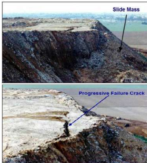
Fig. 2: Failure of Hiriya Landfill (Israel).
