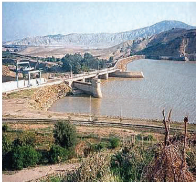
Fig. 1: Fergoug dam (Algeria).
