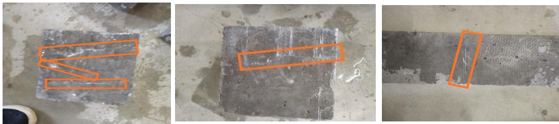
Fig. 16: Healing of cracks in cube and beam samples.
