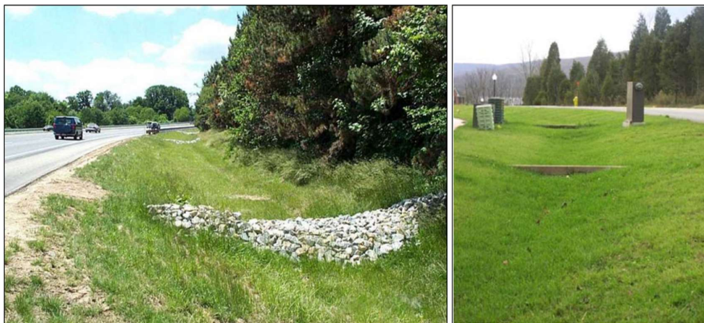
Fig. 5: Enhanced grass swales feature check dams that temporarily pond run-off to increase pollutant retention and infiltration and decrease flow velocity.
