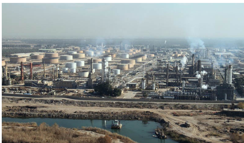
Fig. 1: Photograph of oil Al-Dura refinery.
