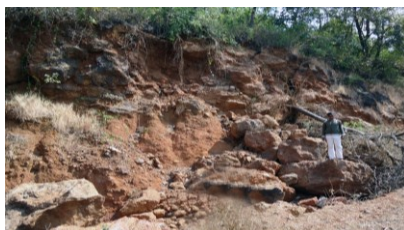
Fig. 12: Rockfall near Bhatgaon – (17°16’ N, 73° 24’ E).
