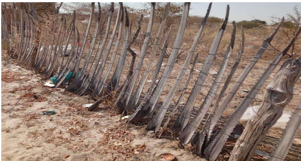
Fig. 20: Waste trapped on a nearby fence. Source: Fieldwork (2025).
