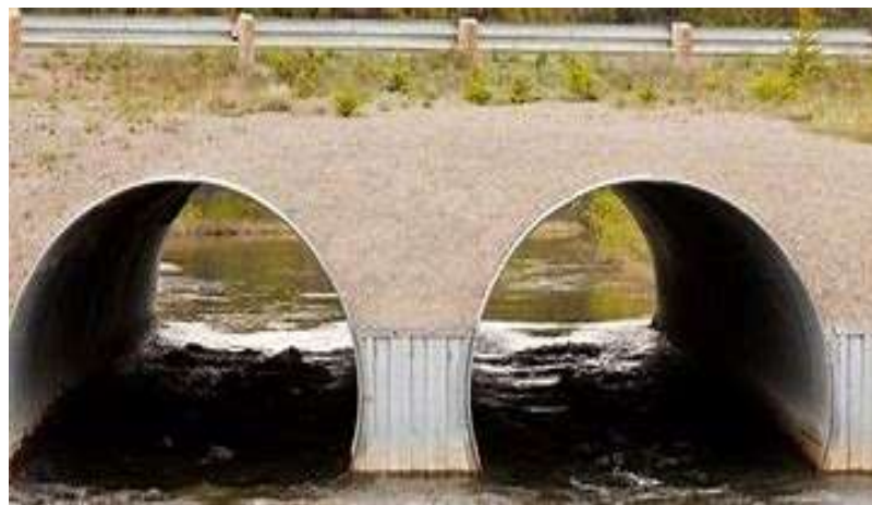
Fig. 7: Culvert under a roadway.
