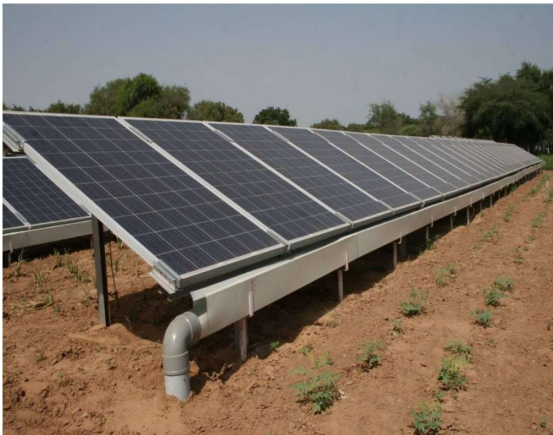
b. AGV system with rainwater harvesting system (Santra et al. 2020).
