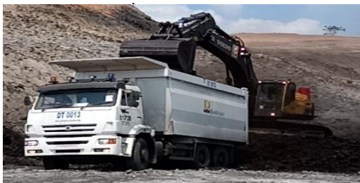
Fig. 2: Dump truck and excavator in Pit 1.
