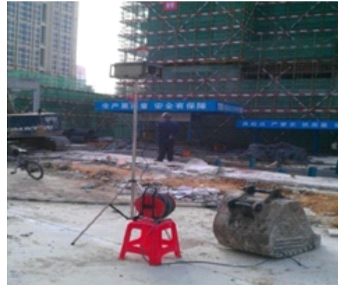
Fig. 8: Test site of project 1.
