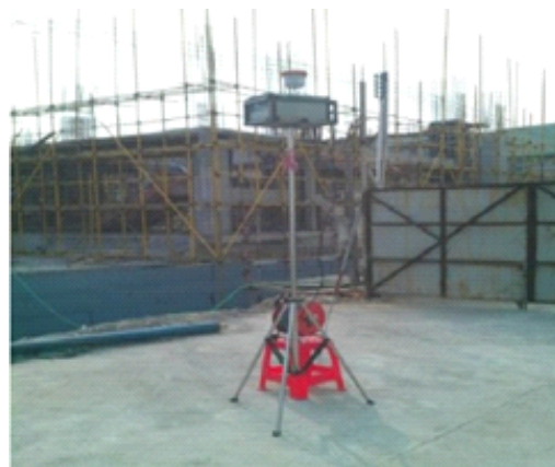
Fig. 9: Test site of project 2.
