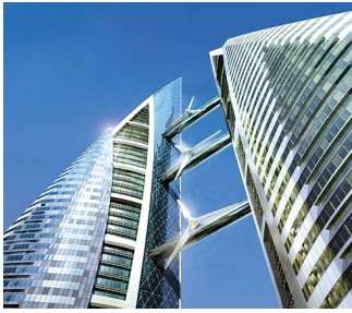
Fig. 7: Bahrain world trade center designed by Atkins- the world's first large-scale building combined wind turbine (picture from Baidu pictures).
