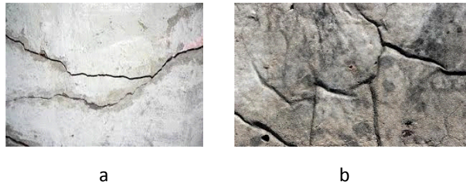
Fig. 8: a. Newly formed cracks, b. Formation of calcium carbonate or calcium hydroxide and healing of the crack.
