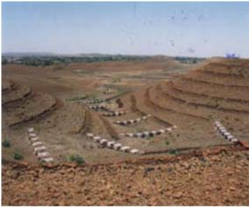
Fig. 1: Terracing and gully-control measures in Jhabua ( http://www.jhabua.nic.in/ )
