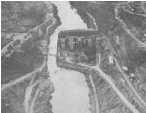
Fig. 1: Works carried out at the WCL site.
