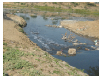
Fig. 4: Effluent channel joins the river.
