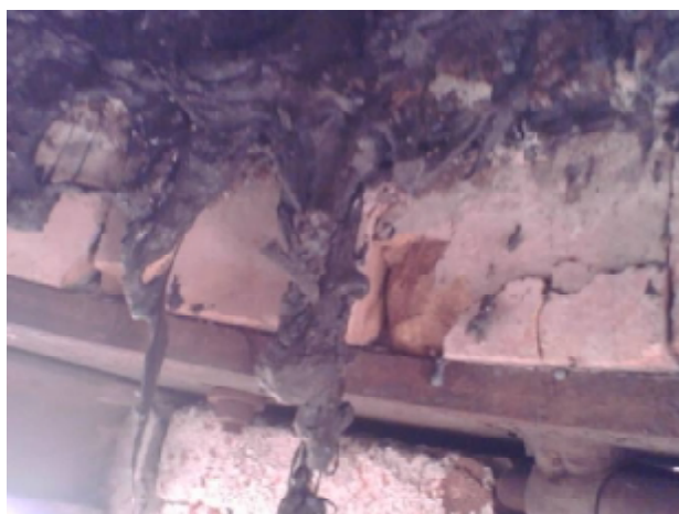
Fig. 3: Broken fire bricks after complete usage.
