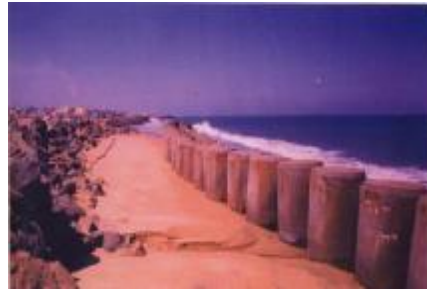
Fig.1: Picture showing the sea wall construction.
