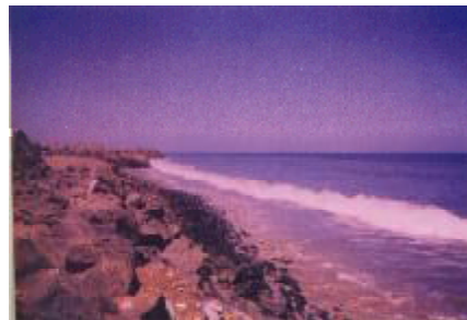
Fig. 2: Picture showing the armour layer of the sea wall.
