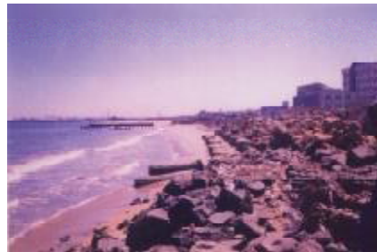
Fig. 3: Picture showing sea erosion remedy wall.
