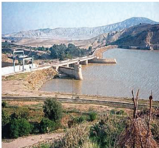
Fig. 1: Fergoug dam (Algeria).
